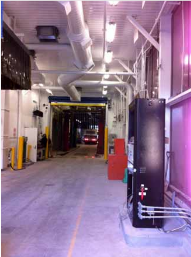
CNG Fueling Bay
