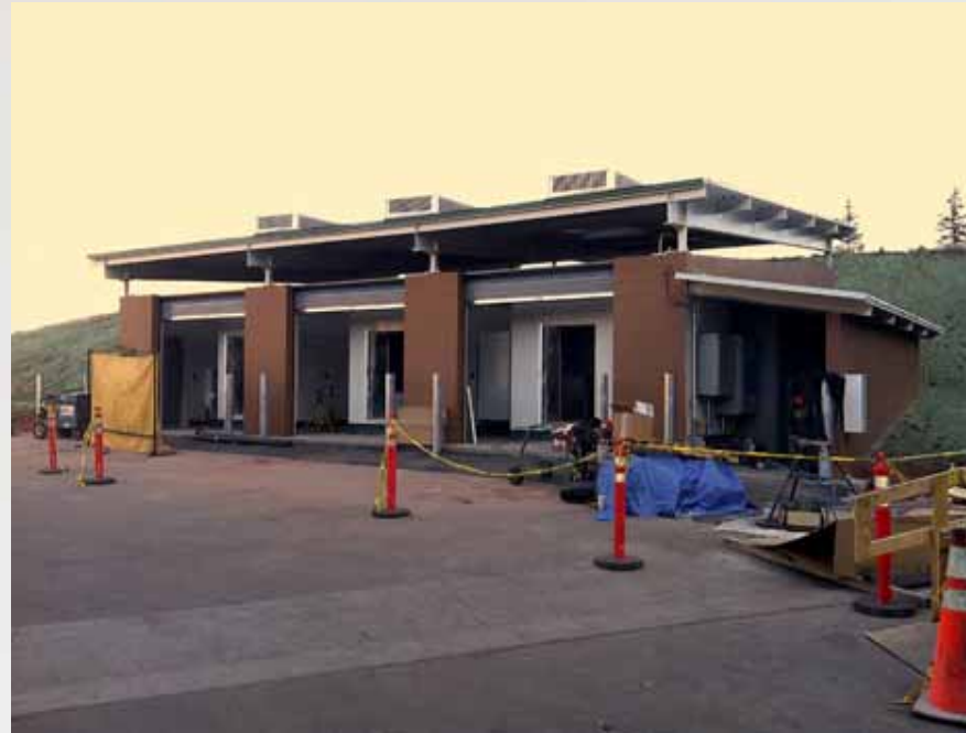
CNG Compressor Station Building
